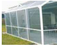
Example of approved design showing support cables
